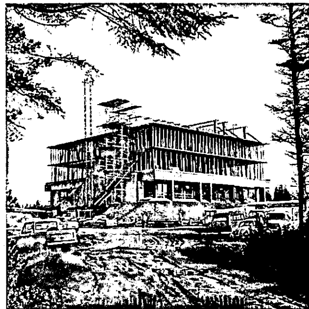
Tioga Hall under Phase IV construction. Three story addition to be completed by fall 1969.
